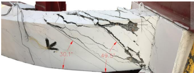
Fig. 8 Specimen C2 failure.
